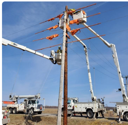
Changing out an electric pole
