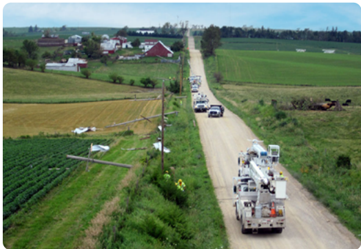
Repairing poles blown down in a wind storm
