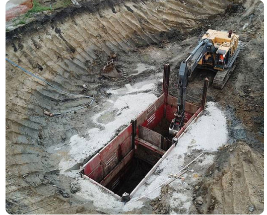
A trunk sewer extension.
