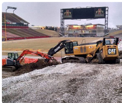
Pump station installation at Jack Trice Stadium at Iowa State University
