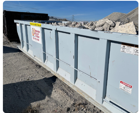
A container holding concrete excess that will be recycled and reused as gravel.
